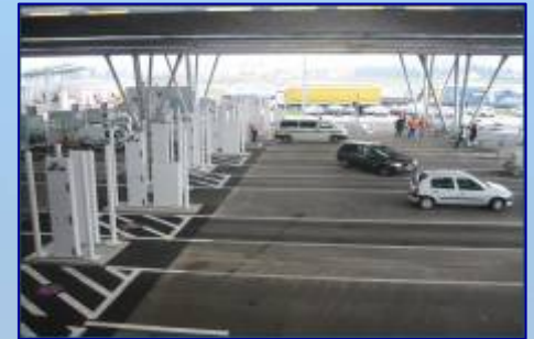
Core installation in Slovenia
